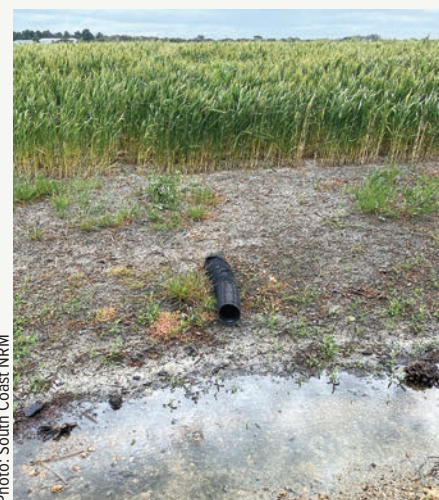
Discharge point of the subsurface drainage system, expelling perched water away from the crop root zone and into an open drain at the Dalyup trial site.
